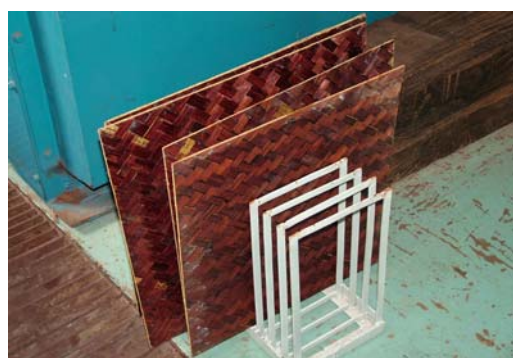
Figure 8. Wall form bamboo mat plywood.
